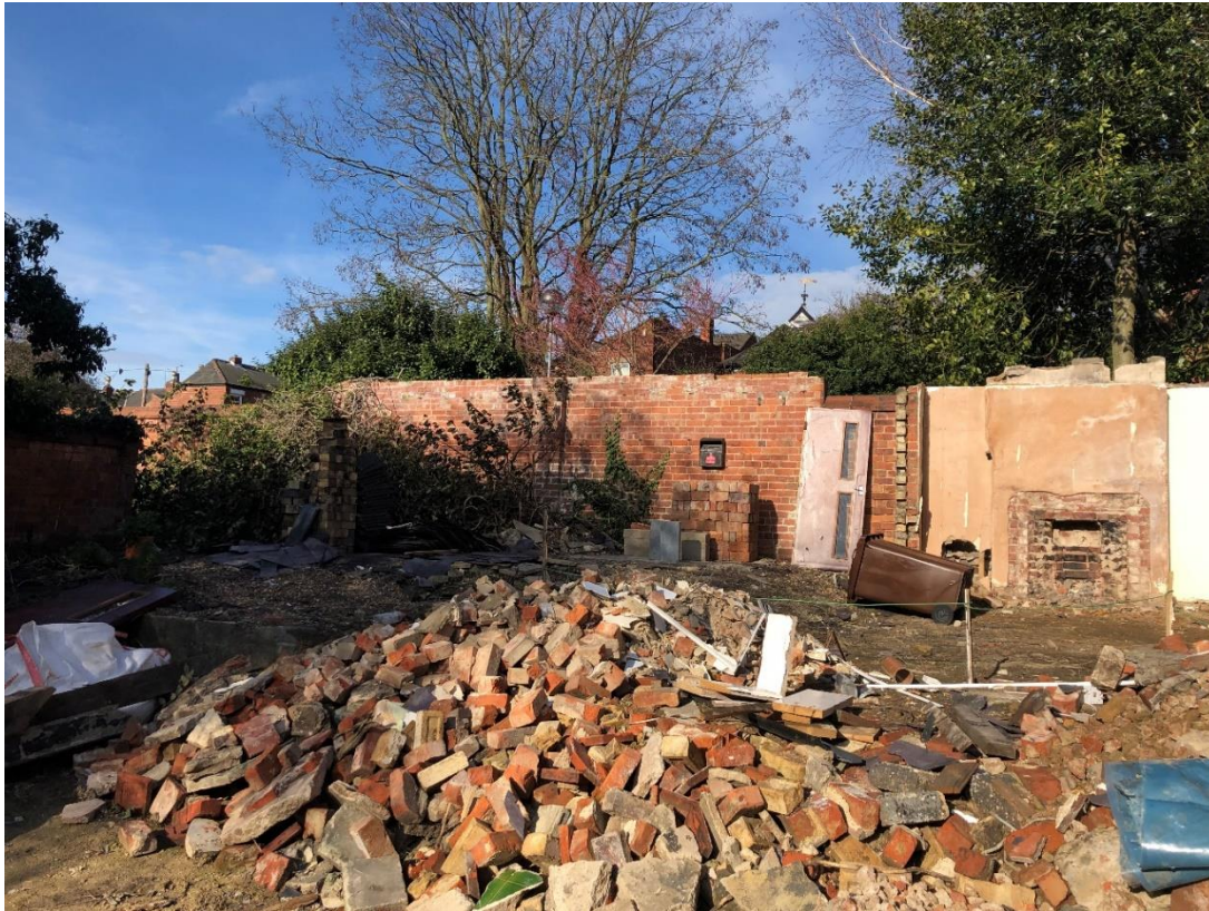
Additional picture of side, north boundary towards the rear of the application site
